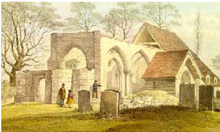
Fig. 3 Restoration work to Leigh Church
