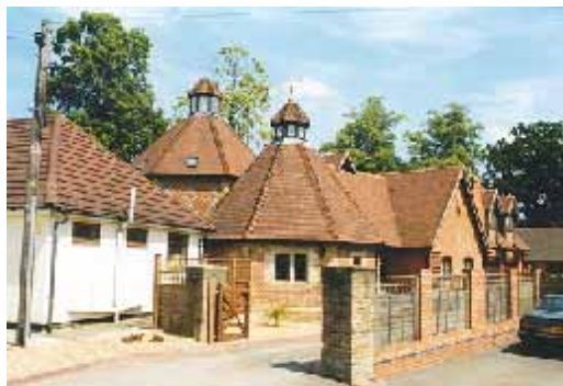
Fig. 26 The Old Waterworks, now a residential property
