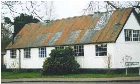
Fig. 35 The Iron Room [ now demolished ]
