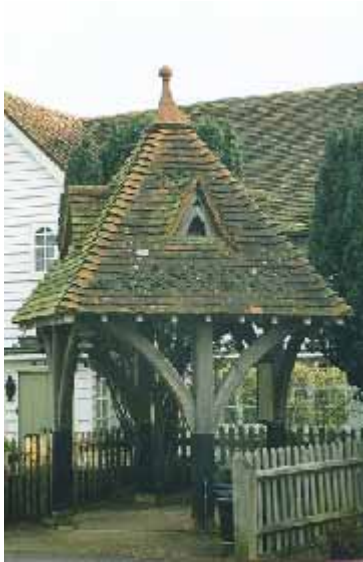
Fig. 33 The Pump House
