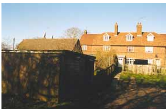
Figure 18 The garages to the rear of Forge Cottages
