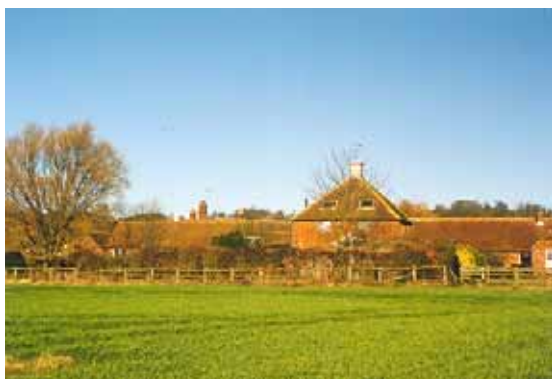
Figure 11 A view north towards the converted farm buildings
