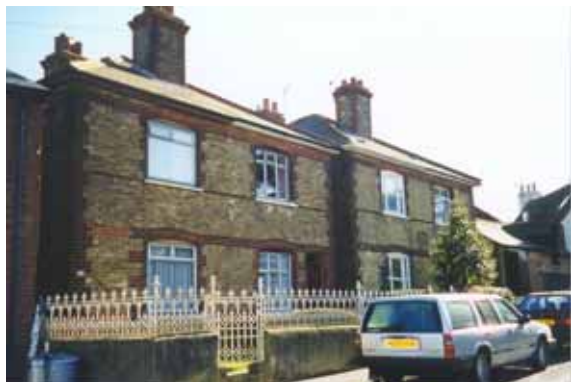
Fig 33: 14 to 20 Station Road
