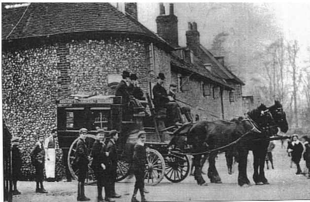
Fig 7: Church Road junction early 20 th Century
