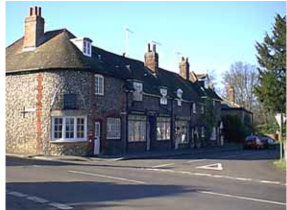
Fig 8: Church Road junction 21 st Century
