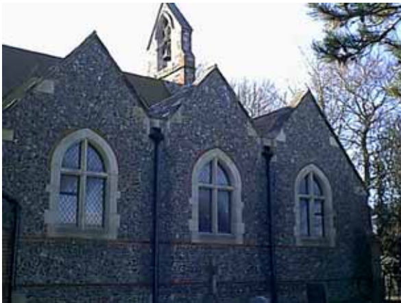
Fig 6: North room extension to St Margaret's Church, Church Road
