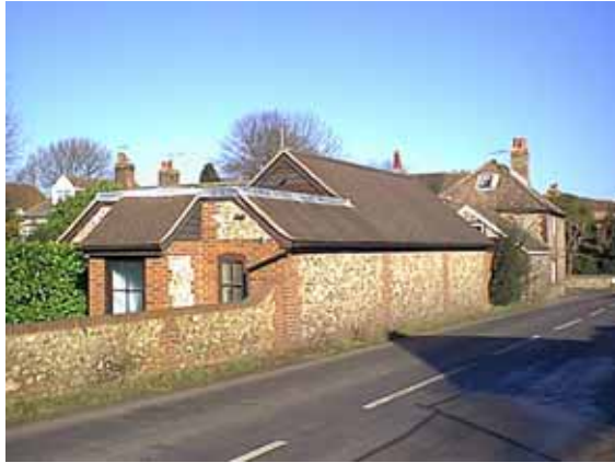
Fig 24 Building to the rear of the Old Post Office, Knockholt Road
