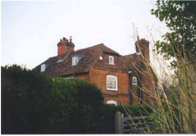
Fig 3: Widmore House Farm, Church Road
