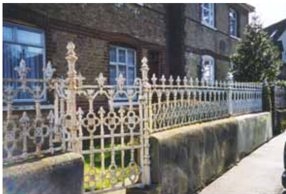
Fig 16: Decorative railings 14 – 20 Station Road
