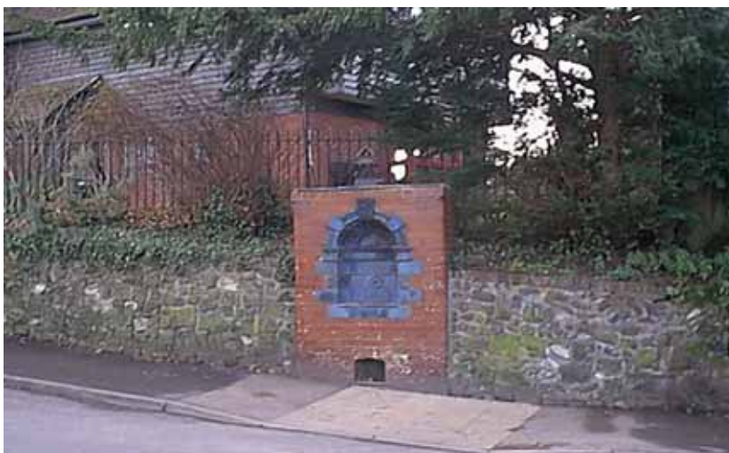
Fig. 23 Glazed brick water fountain, Bower Lane
