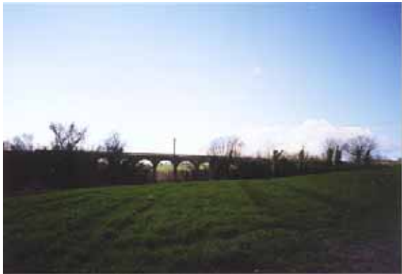
Fig. 22 Railway viaduct to the south west of Eynsford
