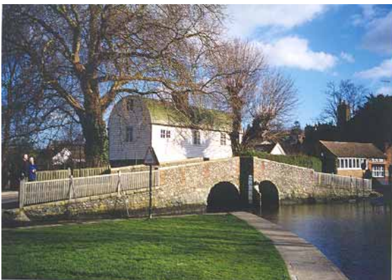
Fig. 7 Old Mill and bridge, Riverside
