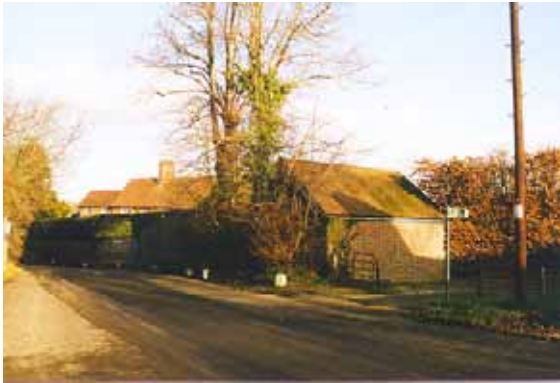
Figure 28 Garage adjacent to The Priors
